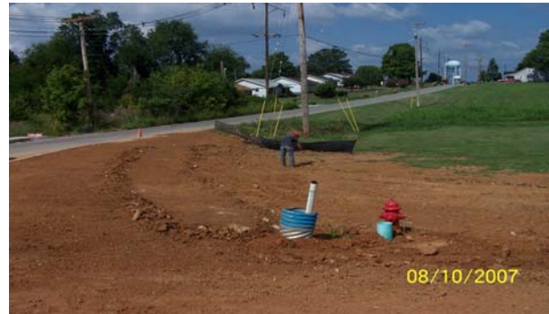
Earth Disturbing work associated with highway maintenance.
